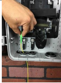
Route Connectorized Feed Cable Through Grommet
