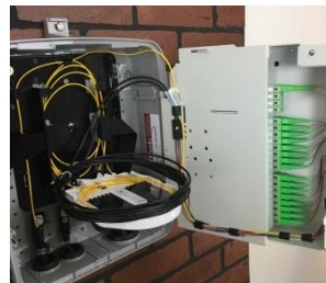
Connect Fibers to Adapters
