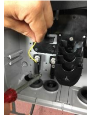
Secure Feed Cable with Hose Clamp
