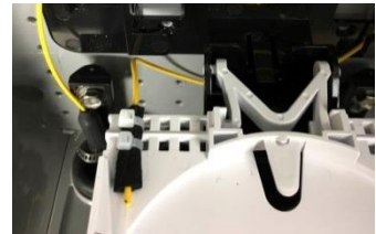
Felt and Cable Ties to Anchor the Buffer Tube
