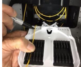
Mark Where Cable Enters the Splice Tray
