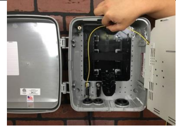
Run Feed Cable Through Grommet
