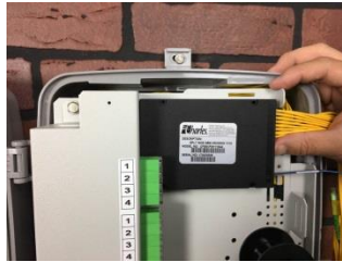
Insert the Splitter
