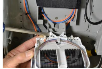
Figure 24 Removing Splice Tray
