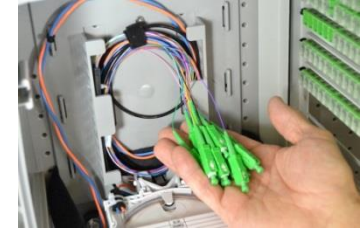
Figure 35 Completed Splice with Connectors Ready to Attach to Bulkhead
