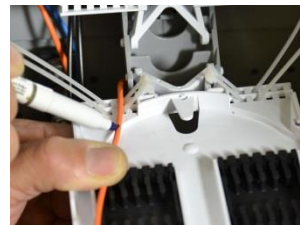
Figure 22 Marking Tube
