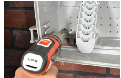
Figure 5 Drill-through Hole
