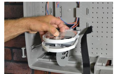
Figure 28 Attaching Tray Cover
