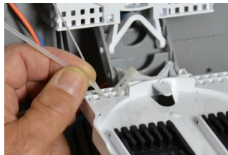
Figure 20 Installing Cable Ties in Left Corner of Splice Tray
