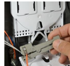
Figure 23 Cutting Tube
