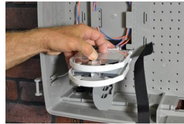
Figure 19 Removing Splice Tray Cover
