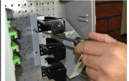
Figure 45 Installing Cable Management Bracket
