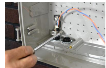
Figure 17 Attaching Hose Clamp
