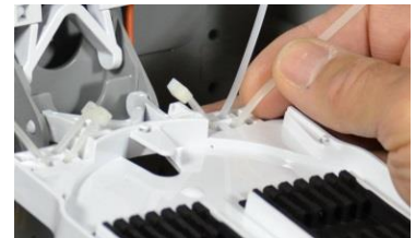
Figure 21 Installing Cable Ties in Right Corner of Splice Tray
