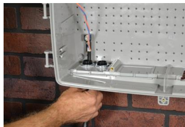
Figure 14 Removing Sheathing to Reveal Buffer Tubes
