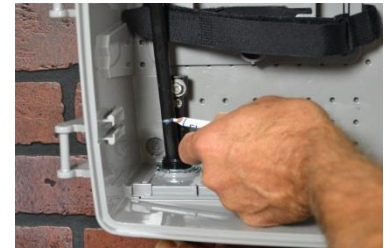
Figure 13 Marking Cut Line on Sheathing
