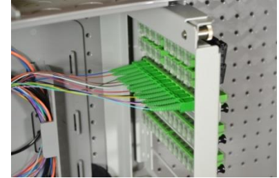
Figure 37 Fanout Connectors Installed in Bulkhead
