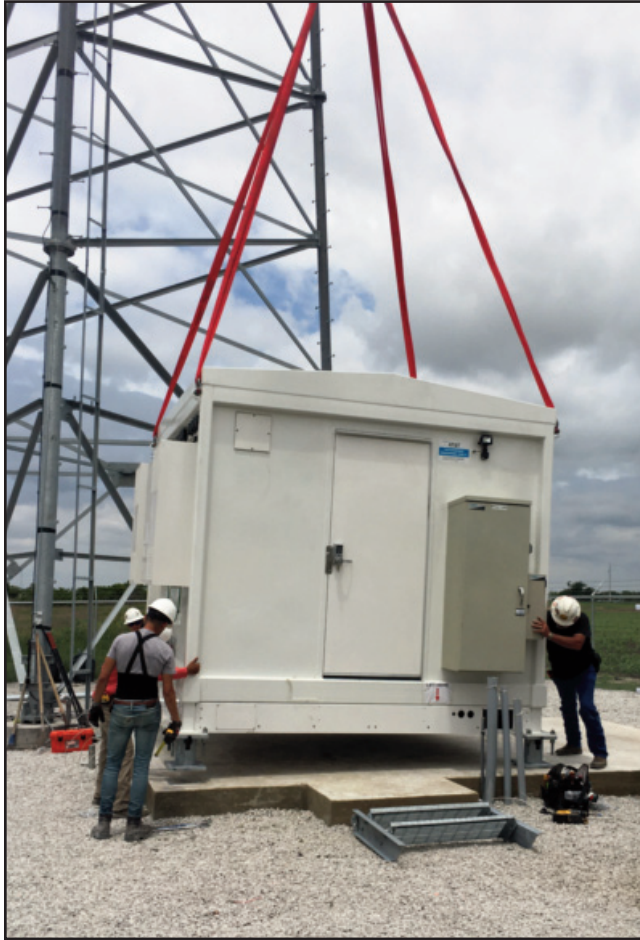
On-Site Crane Installation
