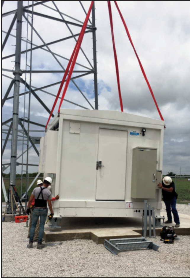
On-Site Crane Installation
