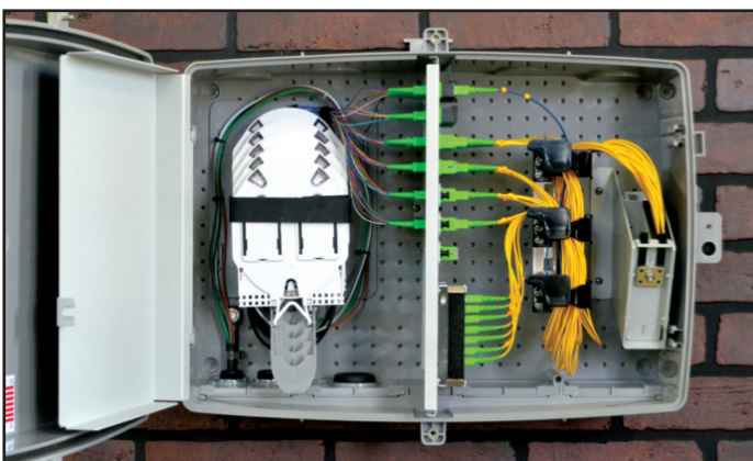
64 Fiber Hub with Splitter Holder and Cable Management
