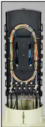
Fiber-Only Drop and Branch Splices (for 6", 8", 10" and 12" diameter pedestals only)
