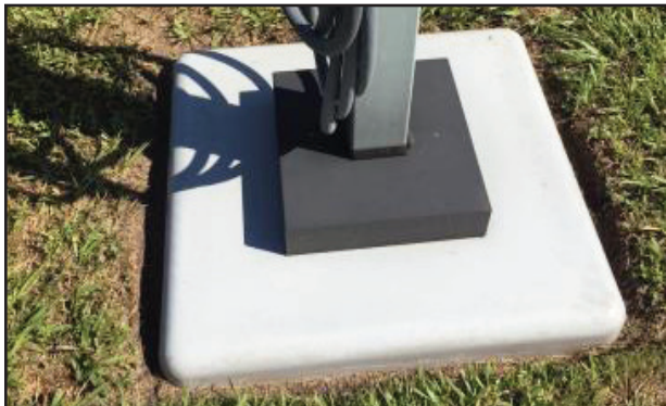
EVC are bolted to CPAD, with workspace below pad
